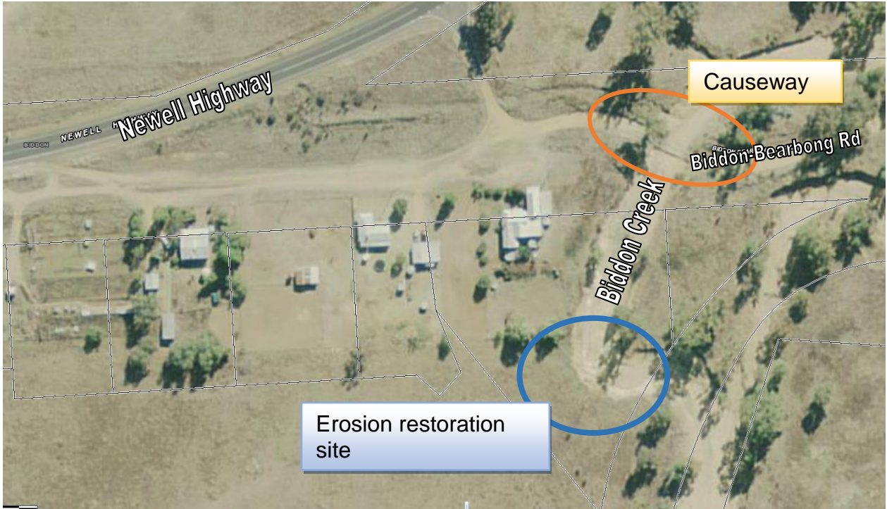
Figure 1: Location of causeway and erosion restoration site – Biddon-Bearbong Rd, Biddon
