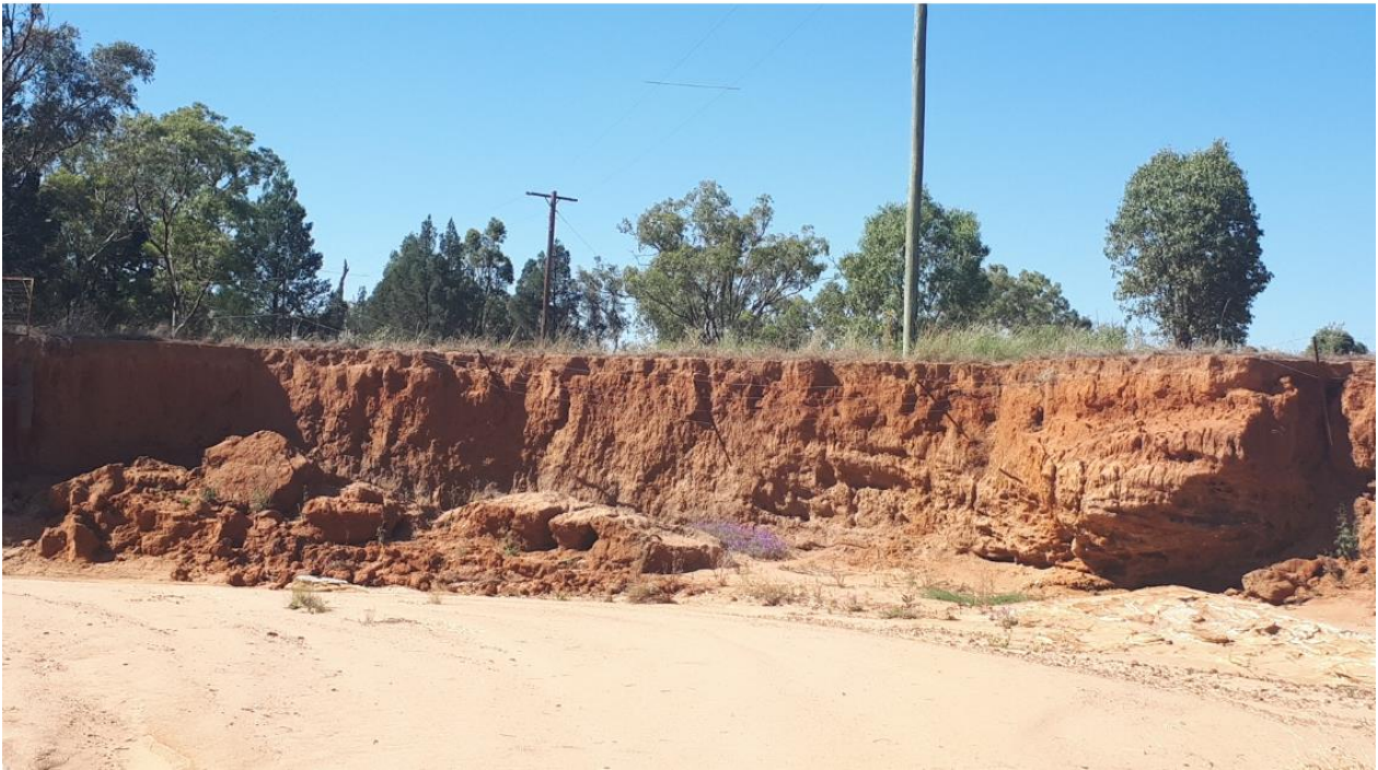
Figure 2: Erosion restoration site downstream of causeway on Biddon-Bearbong Rd
