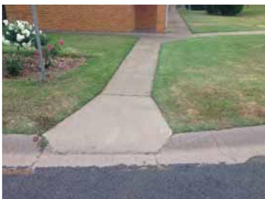
Figure 2.20: Internal road within Cooee Lodge does not have a footpath but there remains a significant lip
