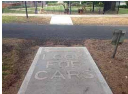
Figure 2.19: Footpath ramps with no kerb lip are desirable
