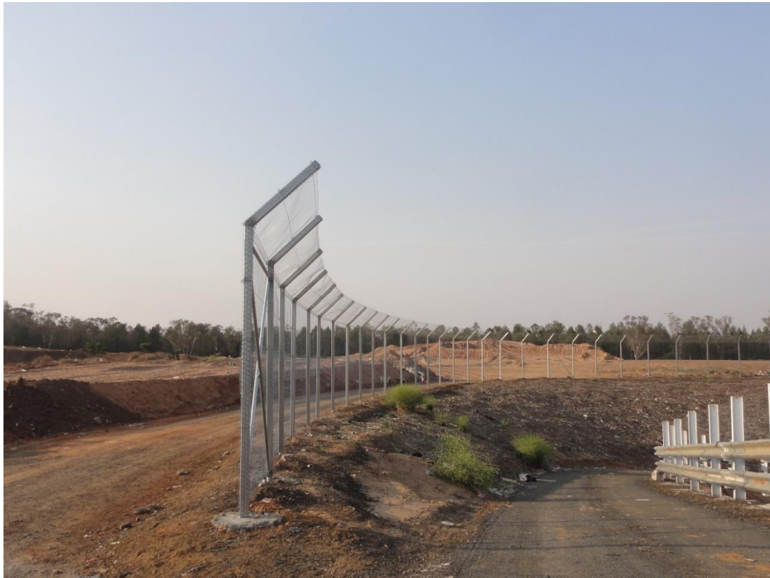
Figure 2: Current litter fence
