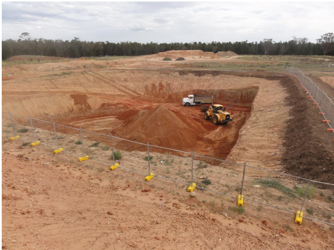
Figure 1: View during construction
