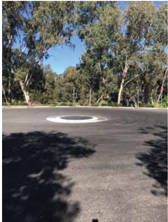
P3 – View towards river across centre of southern roundabout.
