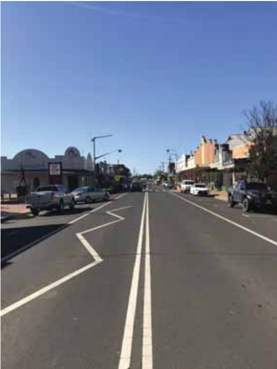
P5 – View north along Miller Street. Marked pedestrian crossing and R3-1A pedestrian crossing signs.
