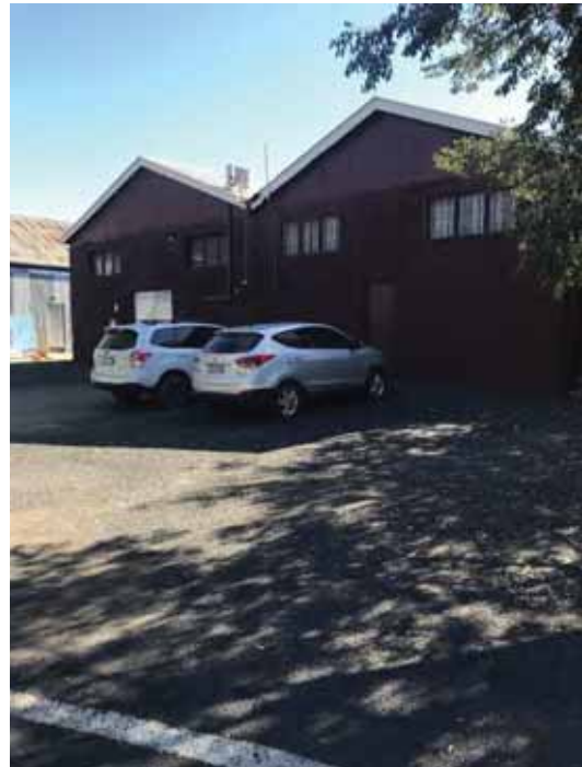
P8 – View of rear of future Library building. 2 or 3 cars normally park there.
